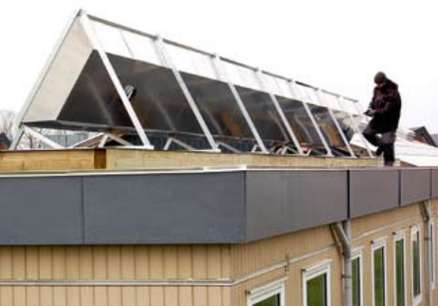
The new industrial models produced by Danish manufacturer SolarVenti provide heating and ventilation for a trade school in Hadsten, Denmark.
